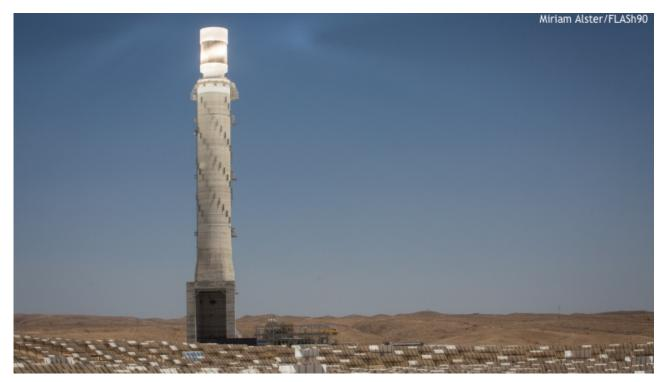
The Ashalim solar and thermal electric power plant in Israel's Negev Desert is up and running. The state-of-the-art facility is equipped with more than 50,000 computer-controlled heliostats or mirrors, which can track the sun in two dimensions and reflect the sunlight onto a boiler placed on top of a tower measuring 240 m-high (787.4 ft). That's higher than some of the tallest sky scrapers in the world and by far the tallest solar tower ever built.
