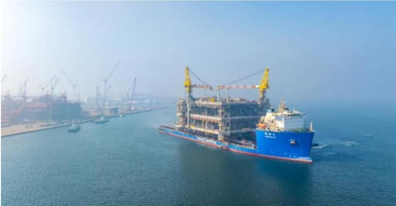
The Marjan oil and gas collection and transportation platform is seen as breakthrough of construction technology of large-scale offshore oil and gas platform for the Chinese builders, weighing more than 17,200 tons, making it one of the world's largest.
